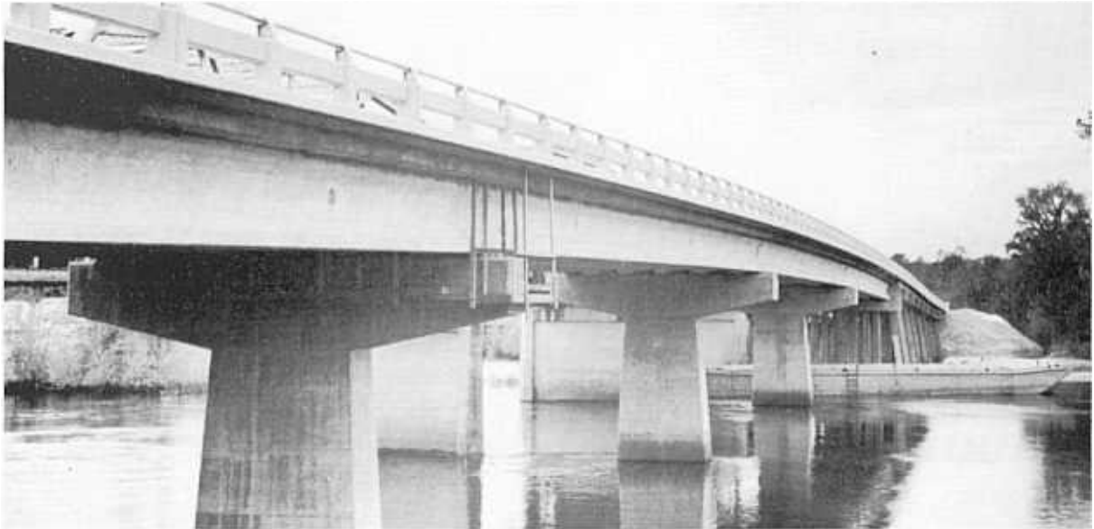
FIGURE 1. CONCRETE WEIGHING LESS THAN 120 LBS. PER CU. FT. PERMITTED 120 FT. SPANS FOR FLORIDA BRIDGE (ENGINEERING NEWS RECORD, JUNE 4, 1964.)
