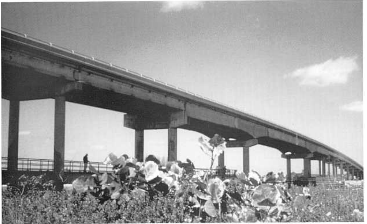
FIGURE 12. SEBASTIAN INLET BRIDGE OVER INDIAN RIVER, FLORIDA.
