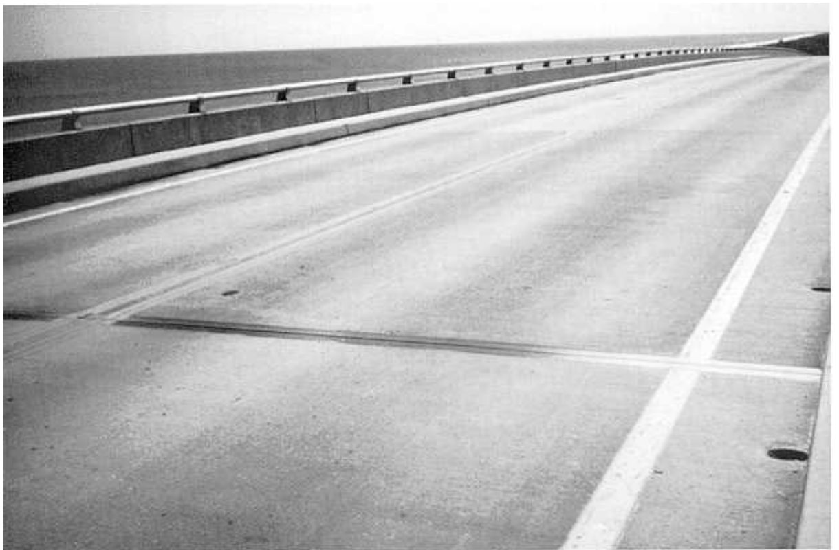
FIGURE 13. EXPOSED WEARING SURFACE, LIGHTWEIGHT CONCRETE BELOW THE JOINT AND NORMAL WEIGHT CONCRETE ABOVE THE JOINT, SEBASTIAN INLET BRIDGE, FLORIDA.
