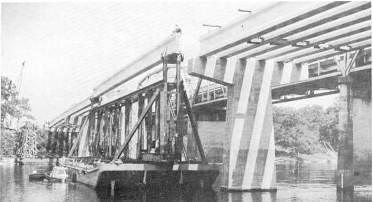
FIGURE 2. BARGE-MOUNTED FRAME PLACED BEAMS. TO THE RIGHT IS OLD TRUSS BRIDGE. BOTH WILL CARRY U.S. 19 TRAFFIC. (ENGINEERING NEWS RECORD, JUNE 4, 1964.)
