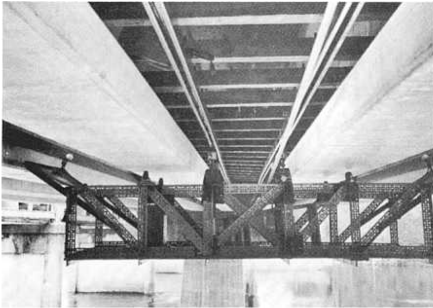
FIGURE 3. SUSPENDED CAR WILL CARRY RESEARCHERS UNDER ONE BRIDGE SPAN. (ENGINEERING NEWS RECORD, JUNE 4, 1964.)
